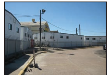
Signal International's buildings after Hurricane Ike. Satellite Shelters provided 22 buildings — the entire complex for Signal's location.
